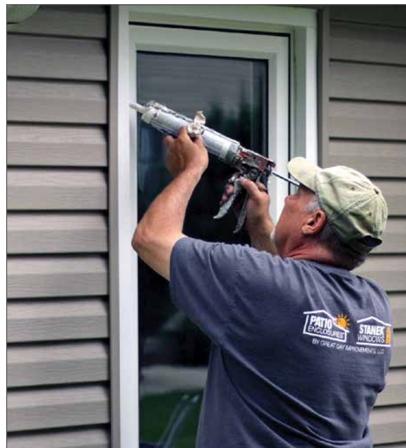
Stanek Windows uses only trained and certified professional installers.
